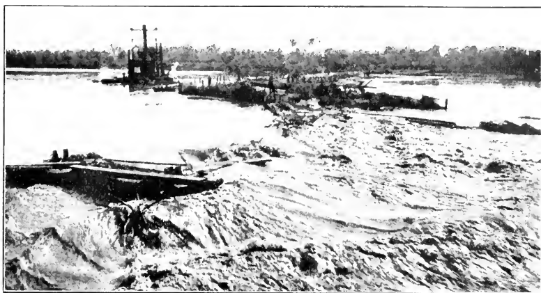
FIG. 7.—HYDRAULIC-FILL DAM, HANLON HEADING, NEARING COMPLETION, SEPTEMBER 4TH, 1915.
